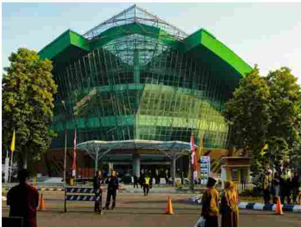
Gambar 1.1 Gedung Auditorium PROJECT ISDB 4 IN 1
